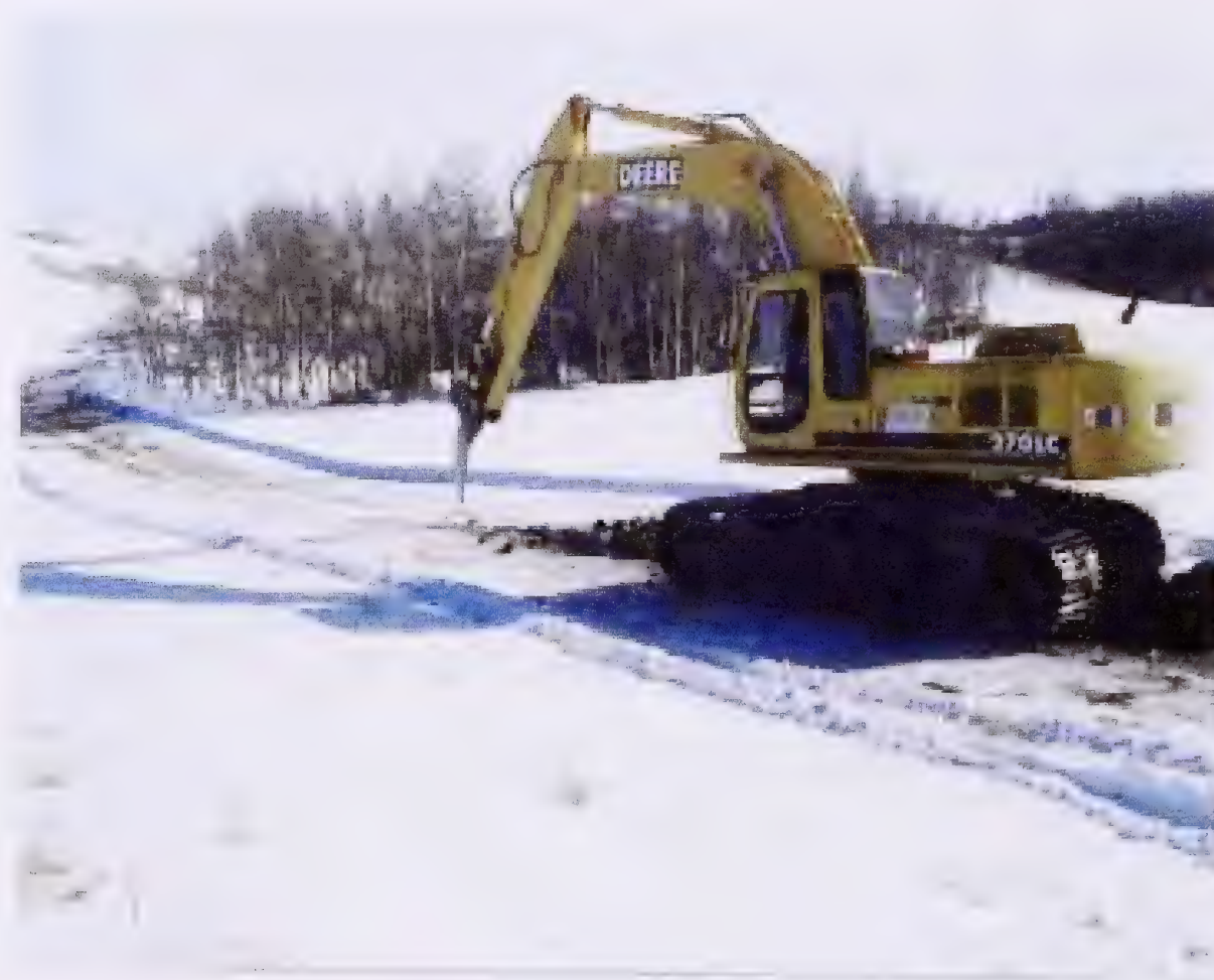
Photo 24 Snow and frozen ground conditions minimize the impact to native prairie vegetation.
